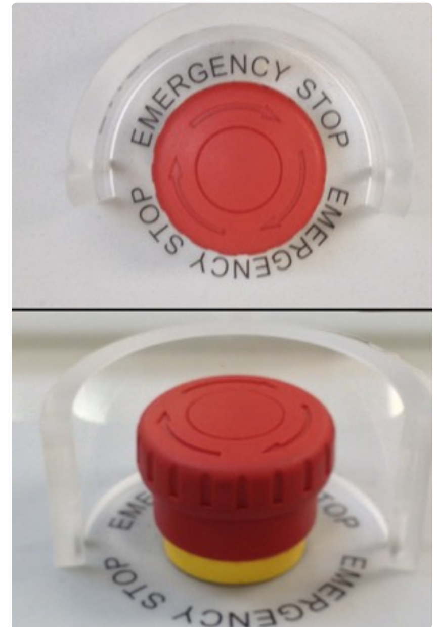
FIGURE 1.4 EMERGENCY OFF (EMO) SWITCH
